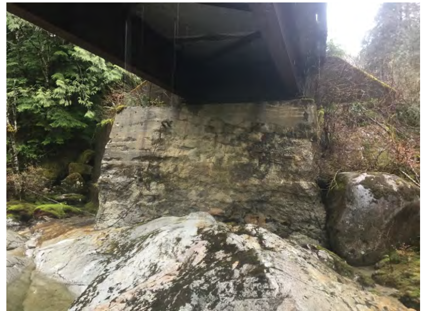
Right Bank Abutment when facing downstream
