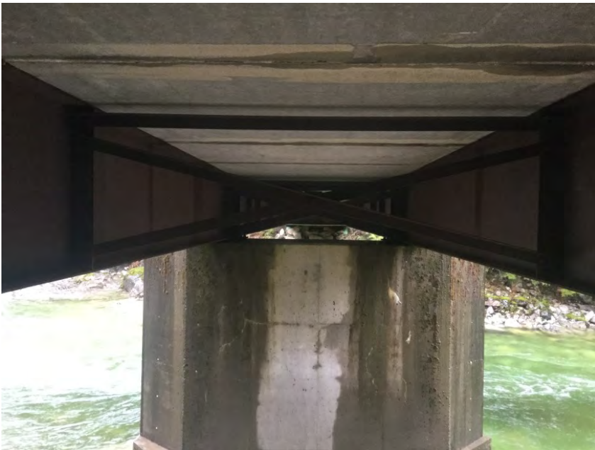
Superstructure - jump span
