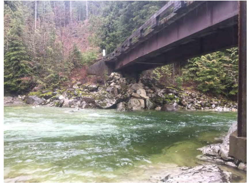
Left Bank Abutment when facing downstream
